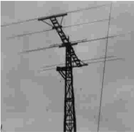
When Les lived in W-S-M, he built this tower. You may be thinking, "That's good, but what's New." I don't know all the details except it is made of timber including the antenna boom. The rotator was home made from aircraft parts
